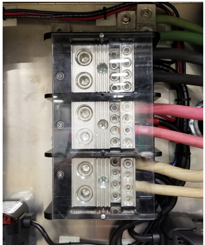
FIGURE 11: TYPICAL SPLITTER BLOCK TERMINATION ▾
