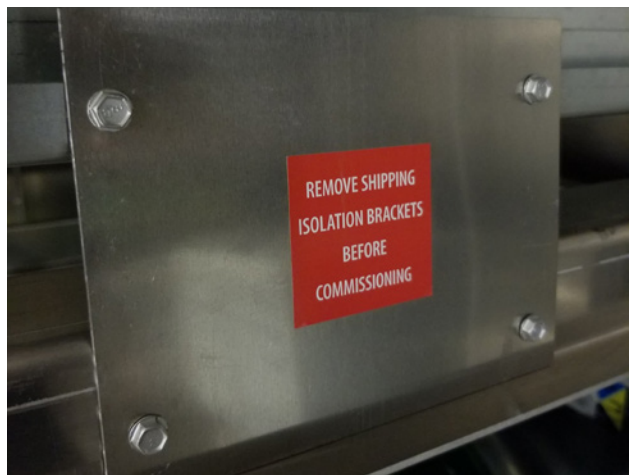
FIGURE 9: TYPICAL FAN BASE SHIPPING BRACKET ▼
