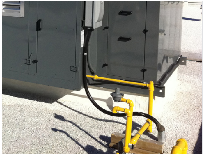
FIGURE 12: ELECTRICAL INSTALLATION W/PITCH POCKET ▼
