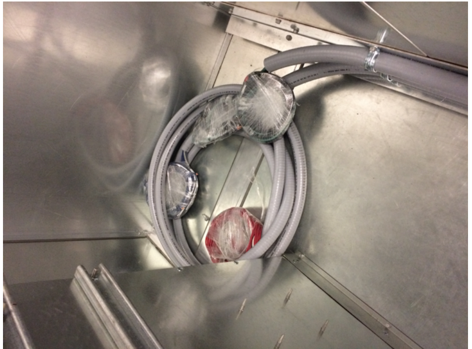
FIGURE 7: HIGH VOLTAGE WIRES SPOOLED ▼
