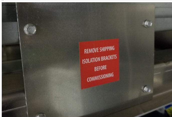
FIGURE 9: TYPICAL FAN BASE SHIPPING BRACKET ▼
