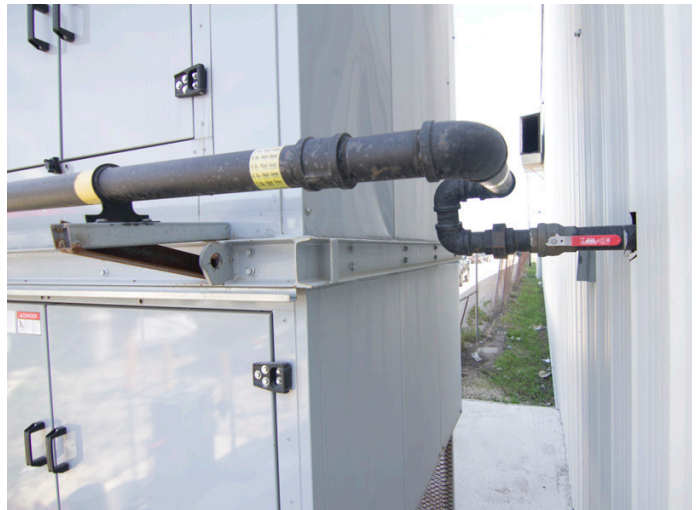
FIGURE 18: TYPICAL GAS LINE SHUT-OFF VALVE ▼
