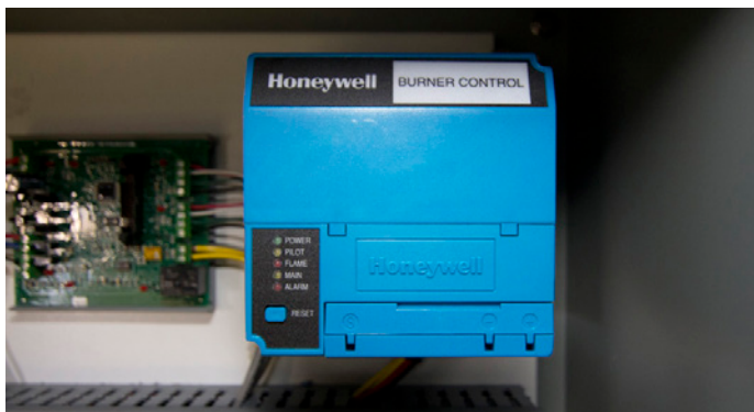
FIGURE 27: FLAME SAFE GUARD CONTROLLER ▼
