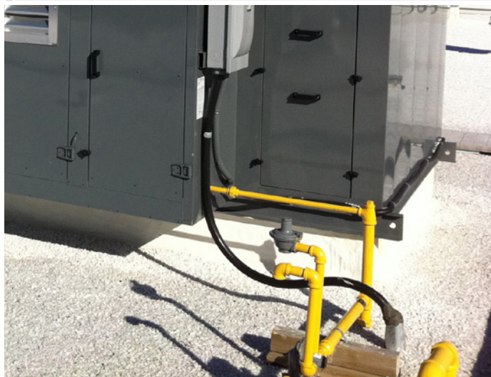
FIGURE 12: ELECTRICAL INSTALLATION W/PITCH POCKET ▼
