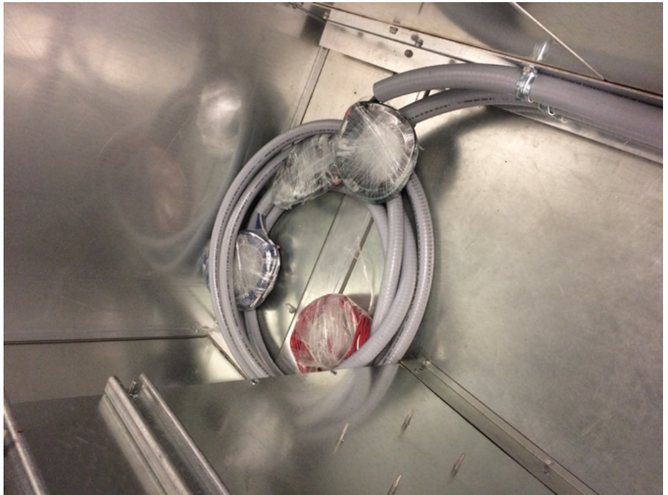
FIGURE 7: HIGH VOLTAGE WIRES SPOOLED ▼
