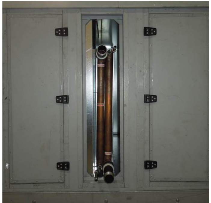
FIGURE 19: UNIT WITH CHILLED WATER COILS ▼
