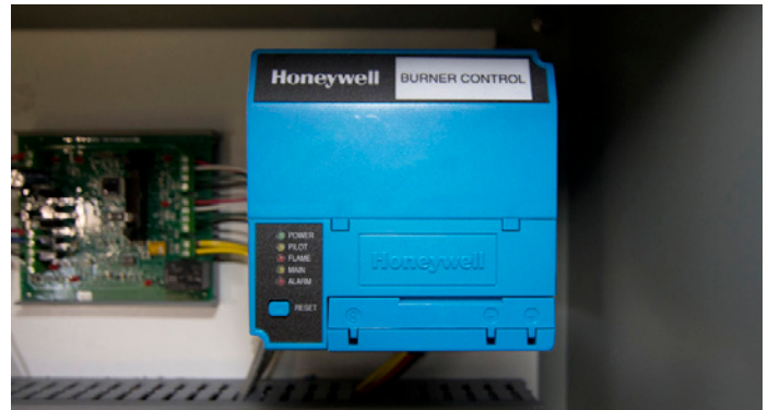
FIGURE 30: PRIMARY FLAME SAFEGUARD RESET ▼
