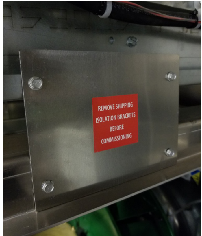
FIGURE 10: TYPICAL FAN BASE SHIPPING BRACKET ▼
