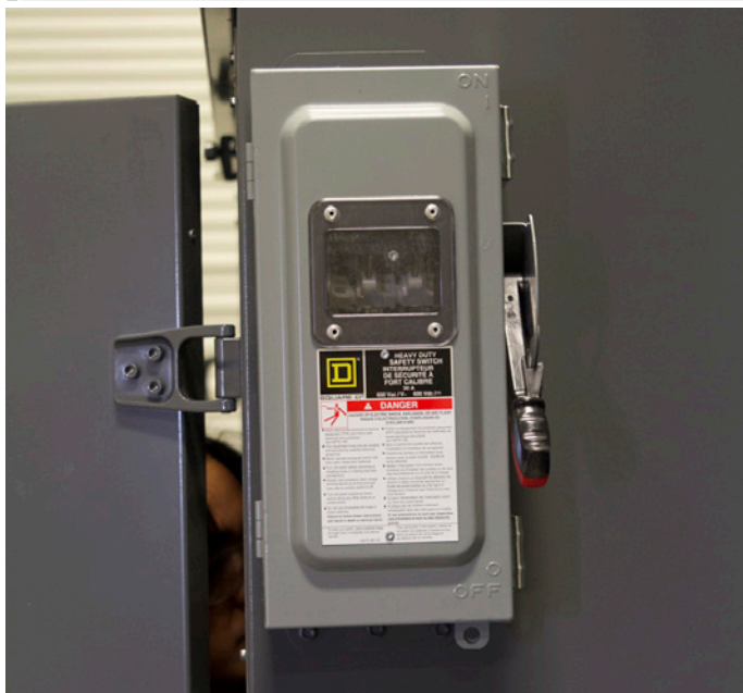
FIGURE 14: TYPICAL FACTORY SUPPLIED DISCONNECT ▼
