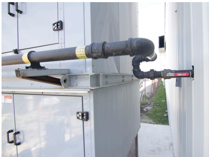
FIGURE 22: TYPICAL GAS LINE SHUT-OFF VALVE ▼
