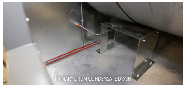
CONDENSATE DRAIN THROUGH CASING
