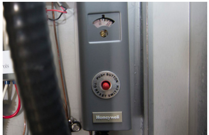
FIGURE 32: LOW LIMIT SAFETY SWITCH ▼
