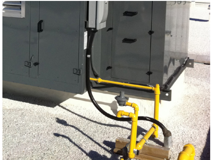
FIGURE 16: ELECTRICAL INSTALLATION W/PITCH POCKET ▼
