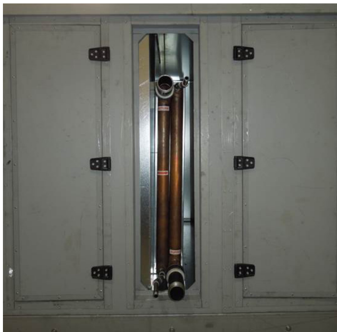
FIGURE 24: UNIT WITH CHILLED WATER COILS ▼
