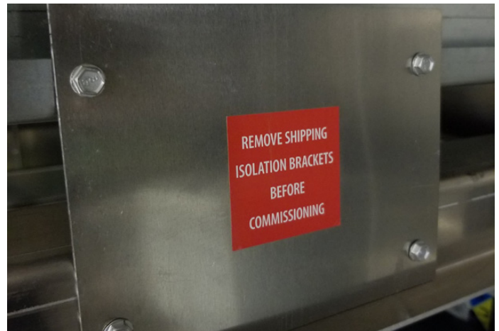
FIGURE 6 – TYPICAL FAN BASE SHIPPING BRACKET ▼
