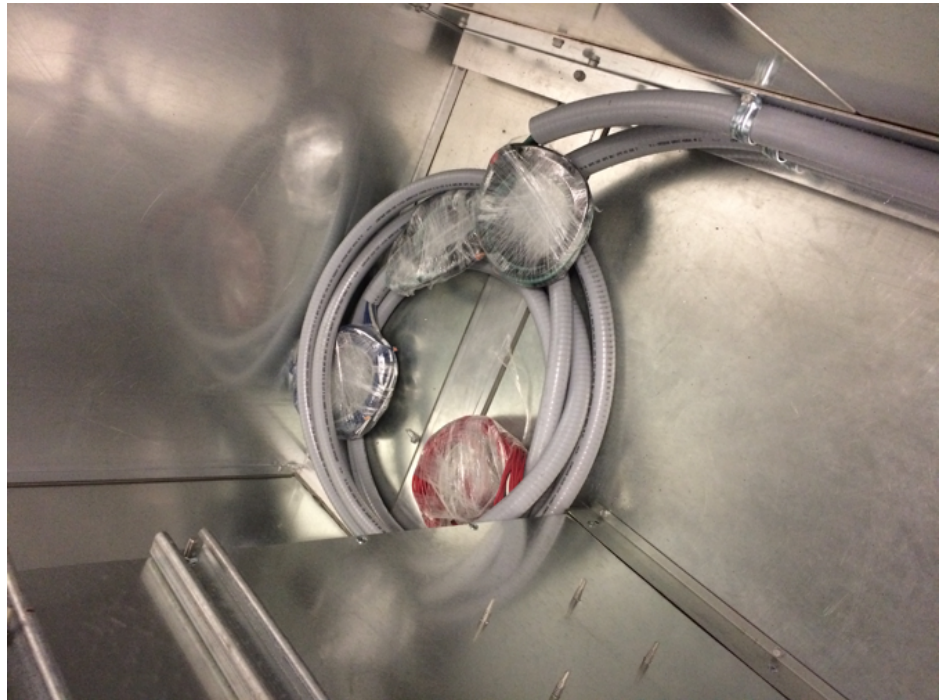
FIGURE 7: HIGH VOLTAGE WIRES SPOOLED ▼
